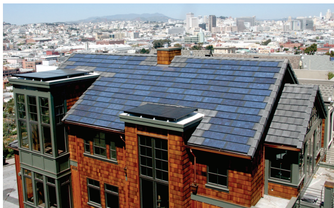
A residential installation of Applied Solar's Building Integrated Photovoltaic (BIPV) roofing tiles.*
